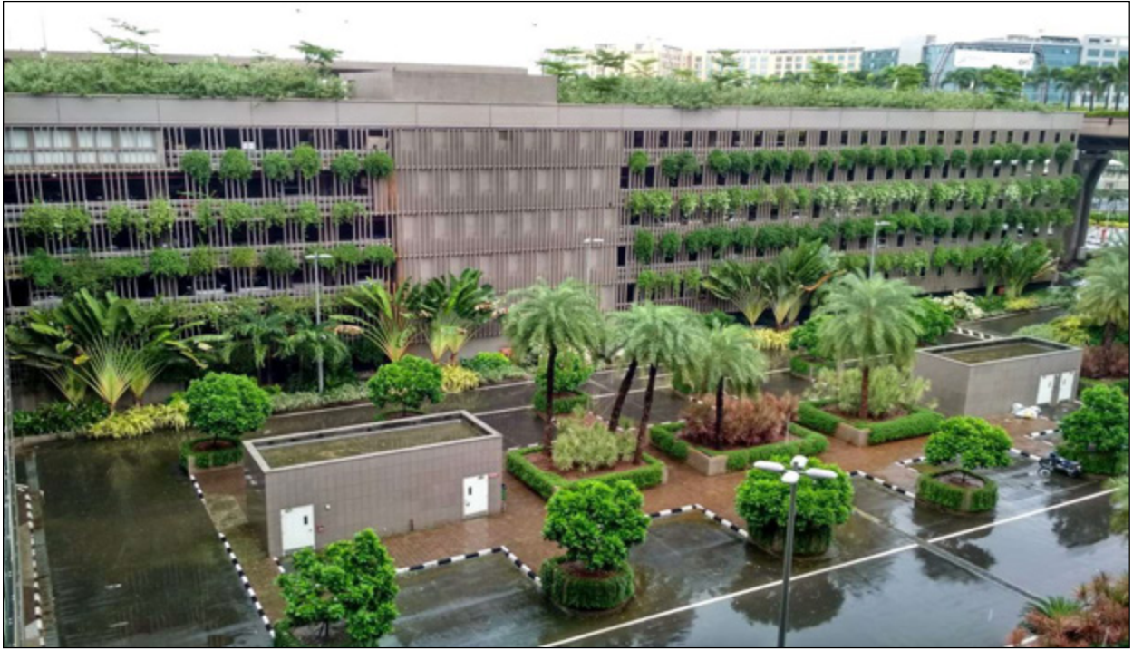
South façade of MLCP & east side landscape at T2, CSMIA
