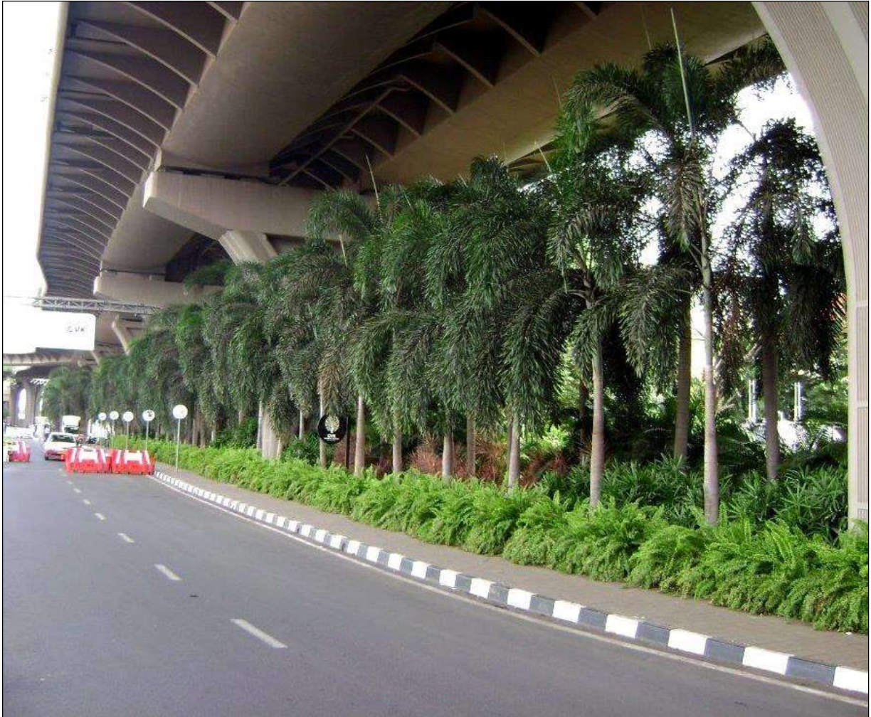
Exit road landscape towards elevated road, CSMIA
