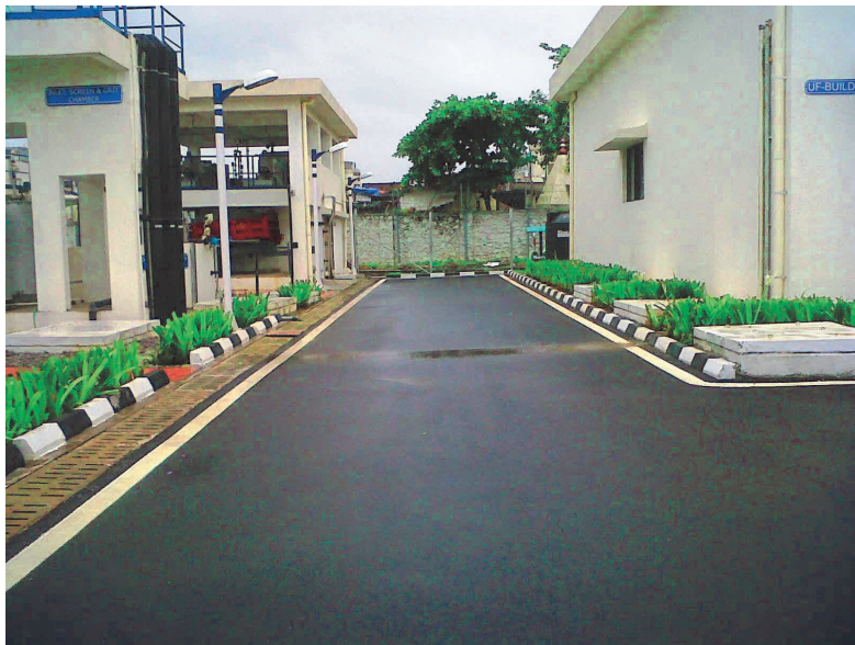
Sewage Treatment Plant @ CSIA
